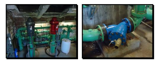
• Replaced failed chemical pump feed line on Micro C pump #1.
