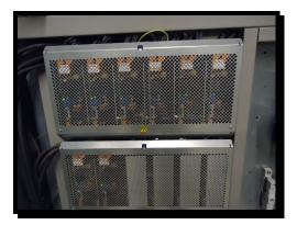
◆ Trouble shot problems with the SCADA system PLC for the blowers and other equipment. Found a breaker tripped and reset systems.
