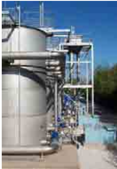
Figure 9-23 Steel Cell BIOSTYR System, Courtesy of Kruger
