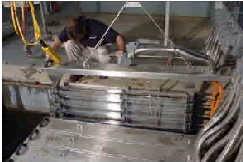
Figure 11-2 Open Channel UV Module Being Removed, Courtesy of Wedeco, ITT Water and Wastewater
