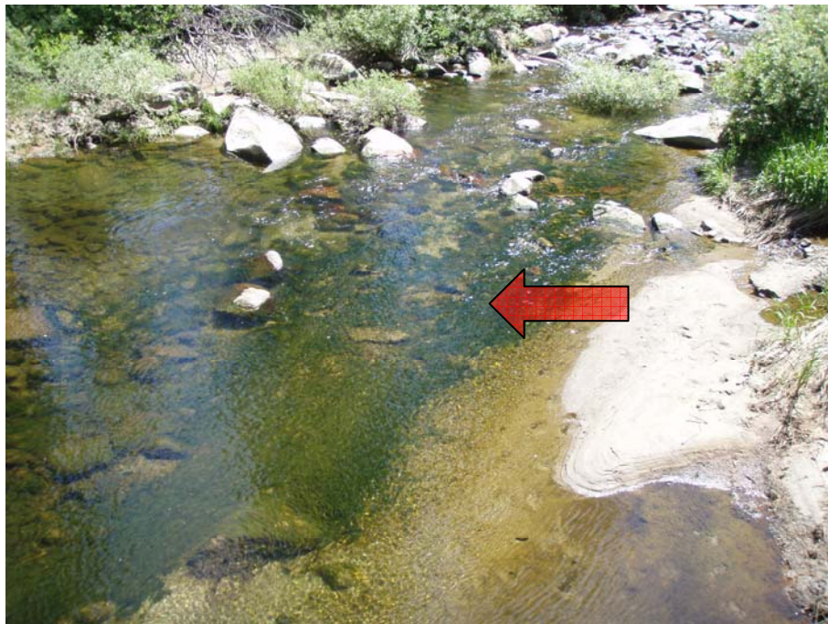
Figure 8. Directly upstream of Towle Mountain Rd, from the bridge. The arrow indicates the approximate sample location. SMJ.
