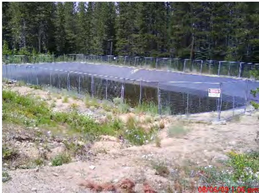
Figure 13 Irrigation Runoff Recovery Pond Located in Northwest Corner of Property
