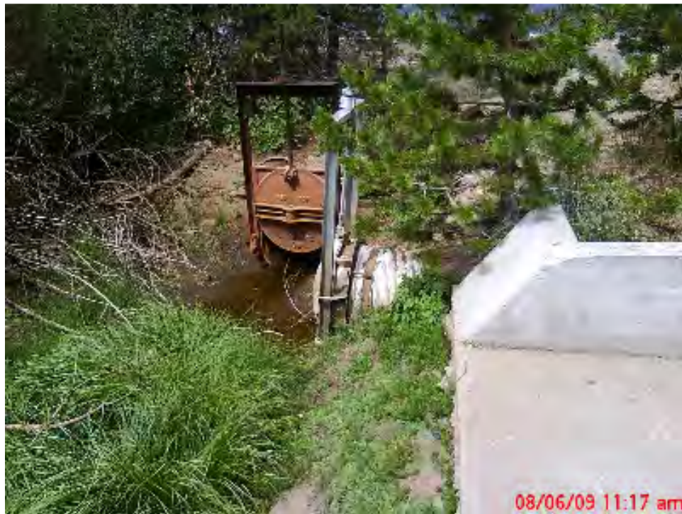
Figure 14 View of Runoff Collection Ditch just Before it Enters Pond (Gate allows Spring runoff of snowmelt to enter an ephemeral stream channel.)
