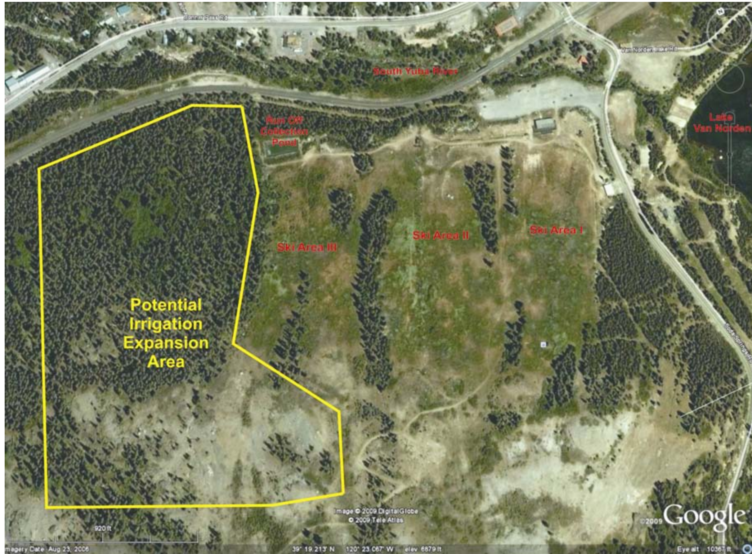
Figure 1 Aerial Photograph of Soda Springs Ski Hill Showing Irrigated Area (Ski Slopes with Darker Green Color) and Surrounding Features
